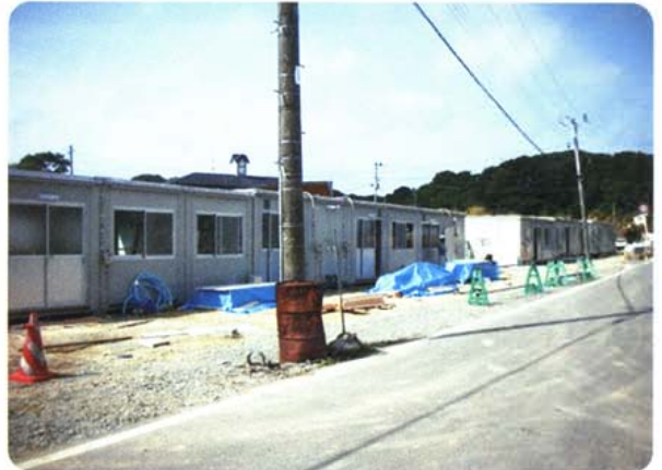
Construction of temporary housing units (residents moved in on July 30)
