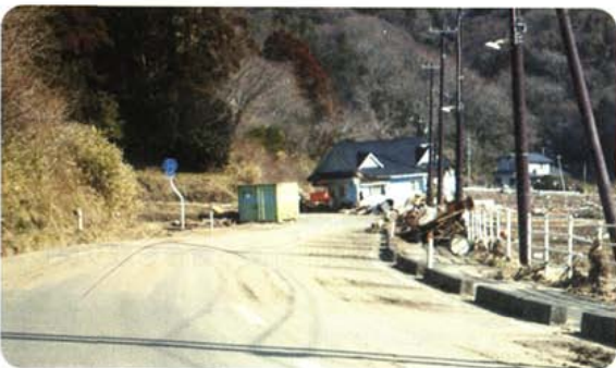
A house dislocated by the tsunami, blocking the road
